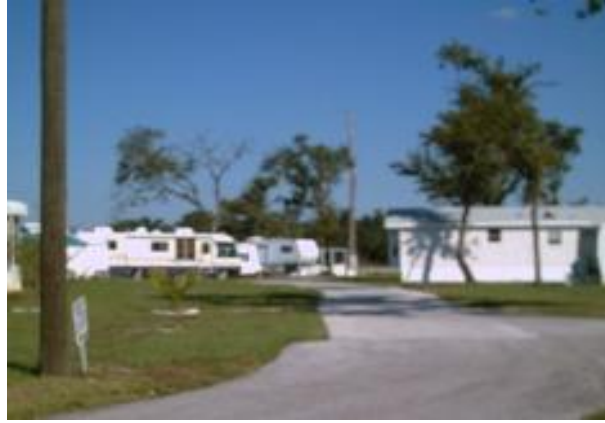
New permanent RV park trailers.
